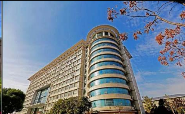
综合楼 ( Comprehensive Building )
